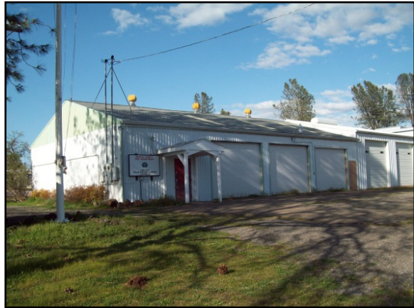
Oak Run Volunteer Fire Department Station
