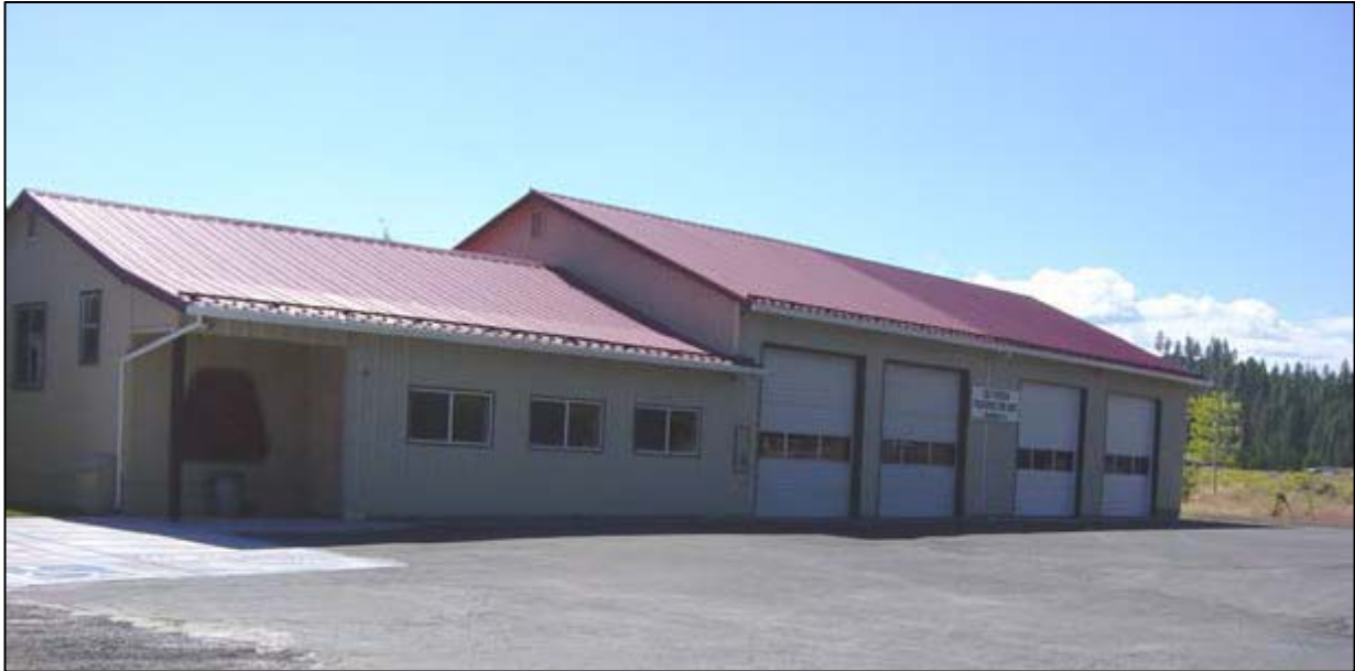
Old Station volunteer firehouse
