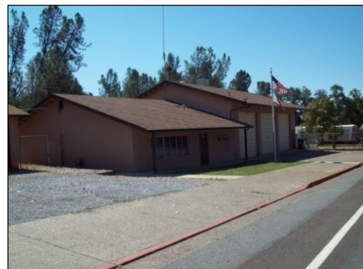
SLFPD Fire Station
