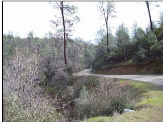
Platina Road – note the large amount of brush and trees to edge of road
