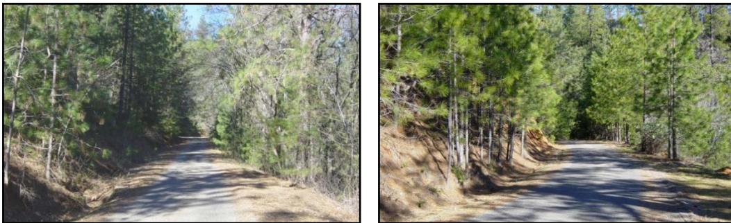
Skyline Drive showing over grown conditions
