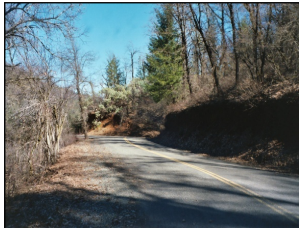
Note brush encroachment on Lower Salt Creek
