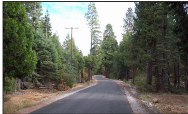
Near Ponderosa Way. Note dense trees and brush up to road edge.
