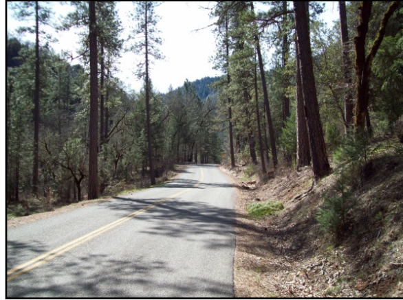
Upper Trinity Mountain Road. Note the brush and trees to edge of road
