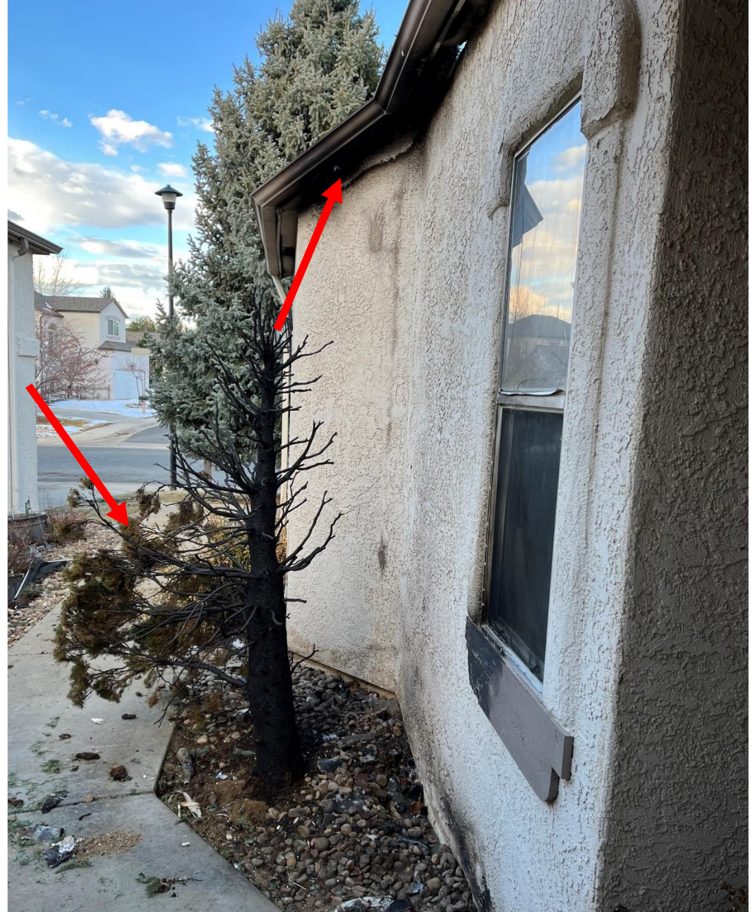
Embers to plant to soffit
